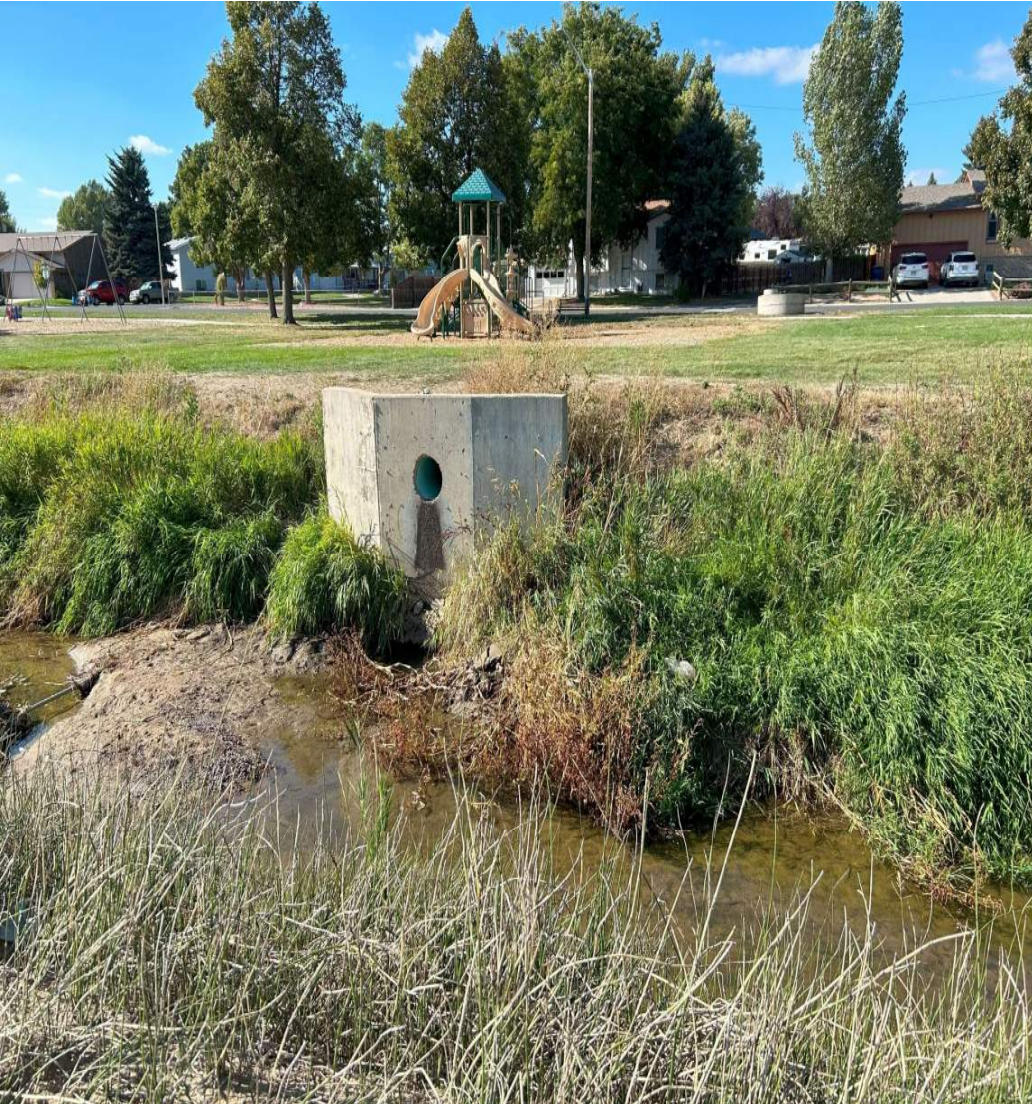
benesch Existing Ditch Connection to the East
