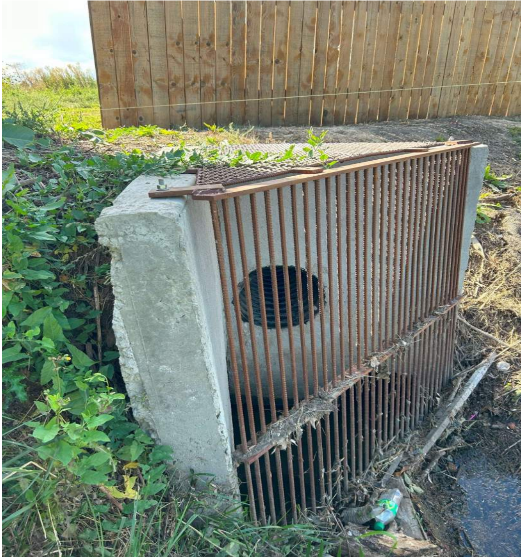
Existing Pond Outlet
