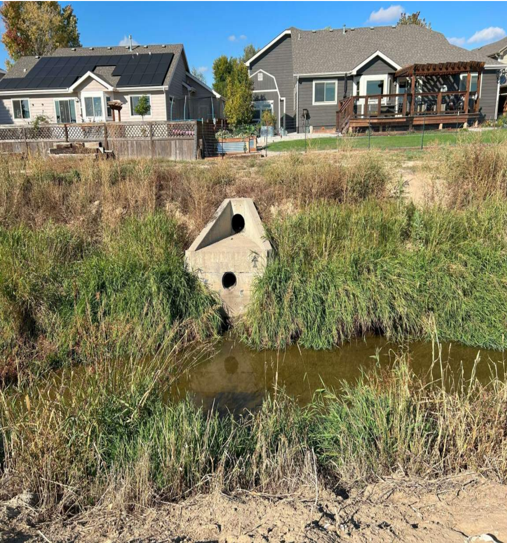
benesch Existing Outfall into Ditch
